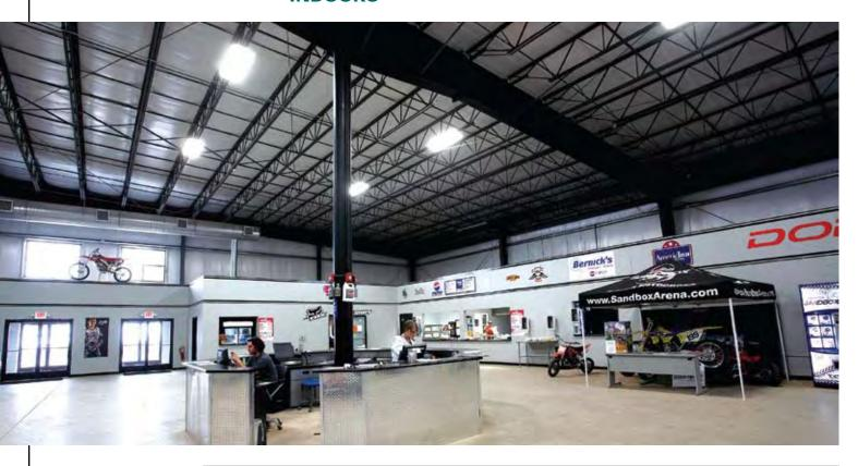
The building's spacious entrance lobby (above) is set off from the rest of the building by darker exterior wall panels (right). The huge building has 6 inches of insulation in the walls and 11 inches in the MR-24® roof system, helping it to stay comfortable inside during the most brutal winter weather.
